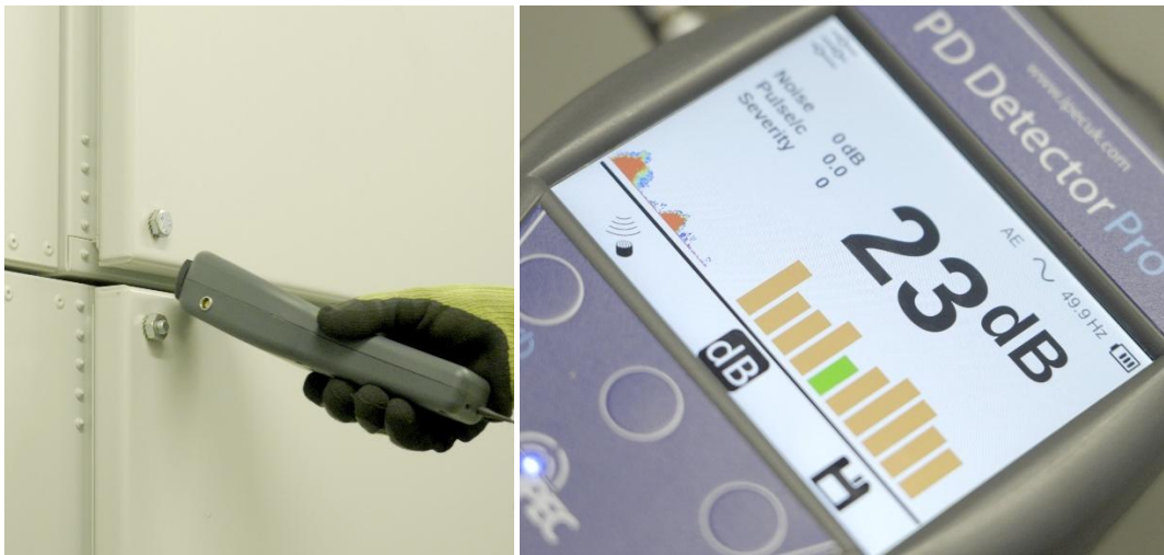
Figure 22 - Photos showing a switchgear panel gap being surveyed in Ultrasonic mode.
